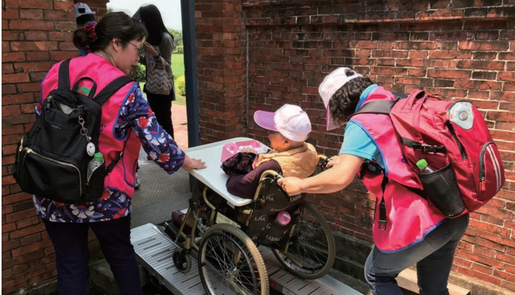
Figure 3: Auxiliary ramps designed and manufactured to overcome height differences in historic buildings, for the use of elderly people with difficulty in walking or those who use wheelchairs.
