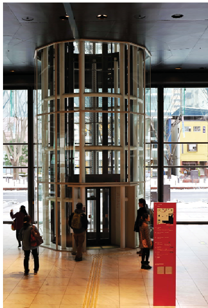
Fig. 8 Tube N° 2, Featuring Elevator Shaft. Note, in this view from inside the Open Square, that the floor is exactly level with the exterior sidewalk. (Copyright: sendai mediatheque)
