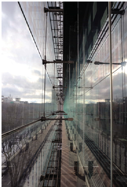
Fig. 9 Double Skin Structure of South Windows. Photograph taken from between the two layers of glass.
