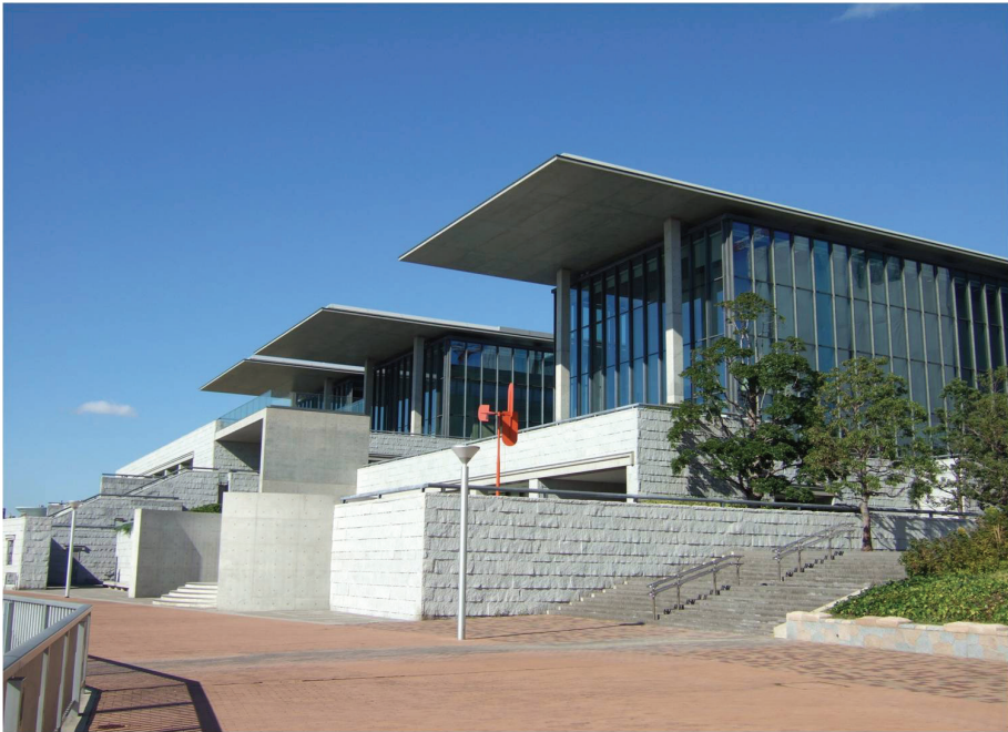
Fig. 8 The new building of The Hyogo Prefectural Museum of Art with Seismic Isolated Structure by Tadao Ando (Copyright: The Hyogo Prefectural Museum of Art)
