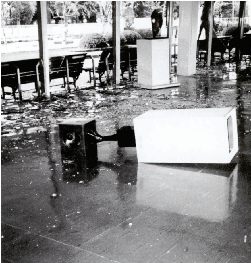
Fig. 3 Exhibition room on the ground floor, The Hyogo Prefectural Museum of Modern Art (Copyright: The Hyogo Prefectural Museum of Modern Art from “Report of Investigation for Museums in the Great Hanshin-Awaji Earthquake I / II”)
