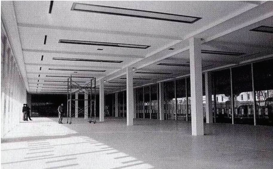
Fig. 2 Slender columns inside the ground-floor gallery, The Hyogo Prefectural Museum of Modern Art (Copyright: The Hyogo Prefectural Museum of Modern Art)
